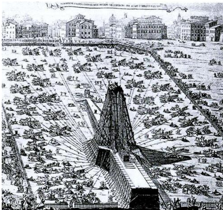
Figure 5 The erection of the Obelisk of Augustus, Saint Peter Piazza, the Vatican. The number and disposition of nine hundred men, seventy-five horses, ropes and pulleys are supposedly portrayed precisely, although the rules of perspective seem to have been somewhat bent in the representation of the buildings in the background.
