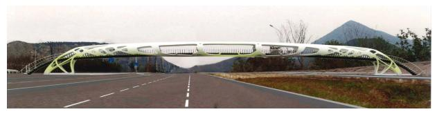
Fig. 1 A footbridge designed using BESO method for Suzhou, China [2].
